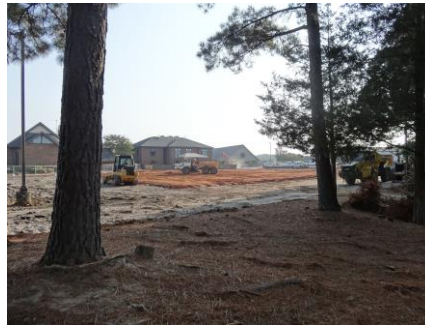
(New building site – Oct 1)
